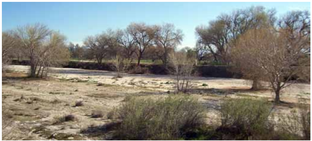
The San Jacinto riverbed near State Street, north of the Ramona Expressway. The proposed elevated road levee would be along existing Record Road, about 1,000 feet north of the Ramona Expressway. Photo by Jenny Gagnon
